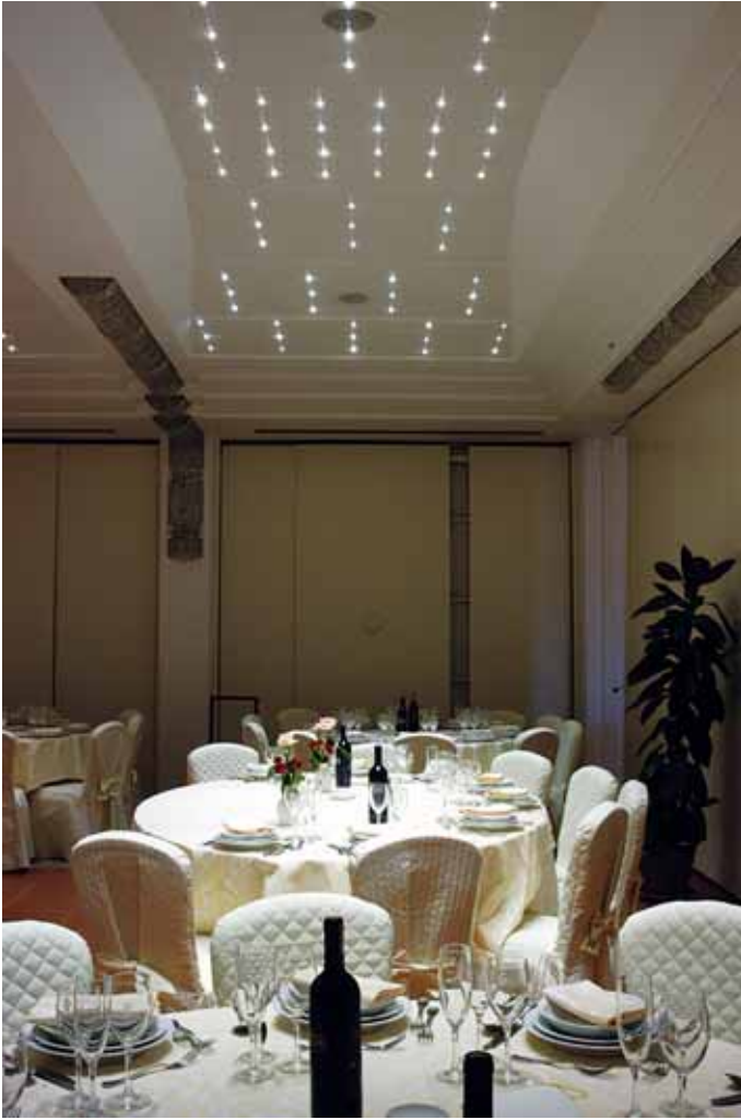
HOTEL GARDEN Siena - Italy Illuminazione salone di 800 mq. Lighting of 800 sqm. n. 51 HIT 150A + n. 1620 quartz glass o.f. diam. 4,3mm. size 12 220 Lux on working plane Project: Arch. A. Bagnoli
